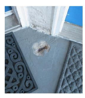
Without proper waterproofing of the surface, these types of spalls will continue to increase throughout the walkways, becoming more numerous over time.
