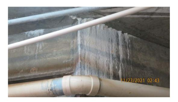
As in the parking decks, these cracks should be sealed to prevent rusting of the reinforcing steel in the slab.
