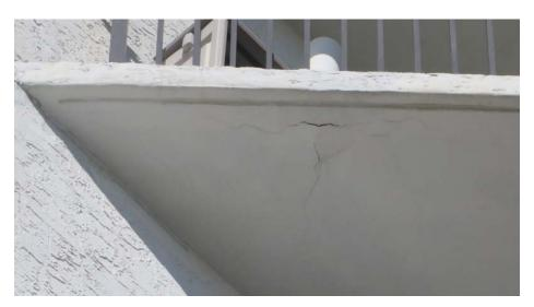
The state of these spalls is such that they can be repaired without extensive demolition of large areas of the balconies. However, without appropriate repairs we have seen where balconies had to be reconstructed.
