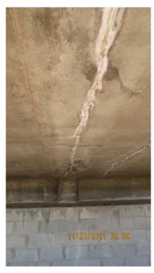
This writer was surprised that the reinforcing steel within the deck had not significantly begun to rust since there was little visual rust seen as part of the laitance (the white residue). It is only a matter of time until this starts occurring. These cracks need to be sealed as part of the waterproof deck coating installation on the deck above. The water coming through the slab is not insignificant as can be seen in the drip lines made in the sand below.
