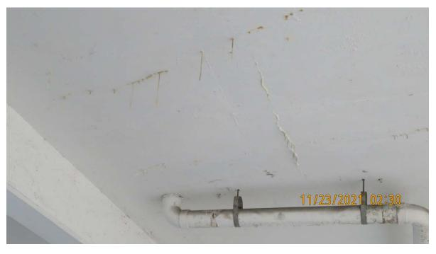
Unlike the cracks in the parking deck where one can see the cracks in the above surface, the pavers of the pool deck prevent seeing the cracks above on its surface.
