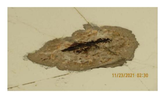
In addition to the spalls there are number of locations where the concrete slab has linear cracks allowing water to penetrate through the deck, similar to what is happening below in the parking deck. These calthemite stalactites are the result of saltwater causing calcium to be leached from the concrete. Over time, this weakens the concrete and leads to the reinforcing steel rusting.
