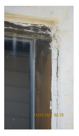
Lastly, the sliding glass doors and windows have single pane glass. The frames are not thermally broken. The glass does not have Low-E coating to reflect the infrared and ultraviolet light from entering through the glass into the unit. Both issues add a significant amount of heat gain in the summer and heat loss in the winter. It is estimated that the cost per unit with new insulated coated glass would reduce the cost of conditioning air by 20% to 30%.
