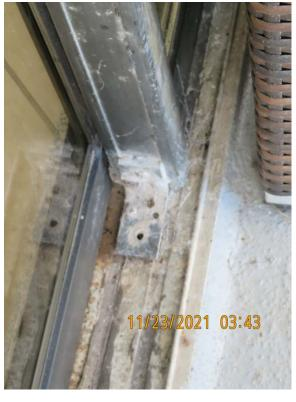
The sealant joints between the aluminum frames and the stucco have deteriorated and broken down. The joints have ceased to operate as a true expansion joint to allow movement between the aluminum frames and the wall.
