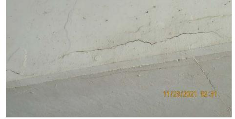
These types of cracks are not uncommon. Sometimes they are the result of water penetrating the girder but most of these appear to be caused by structural movement of the towers above.
