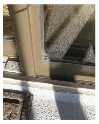
The anchoring hardware connecting the doors to the building has deteriorated and no longer functions as a structural connection.
