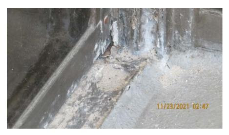
Gaskets between the glass in the aluminum frames have failed.
