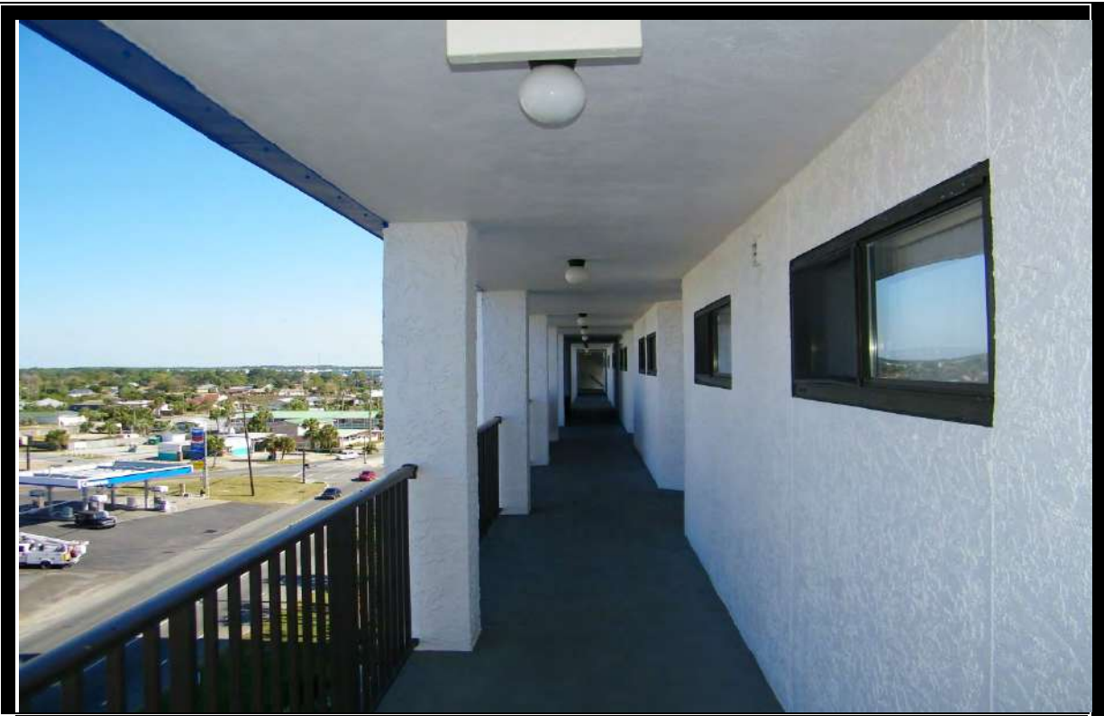
VIEW OF TYPICAL BUILDING COMMON AREAS
