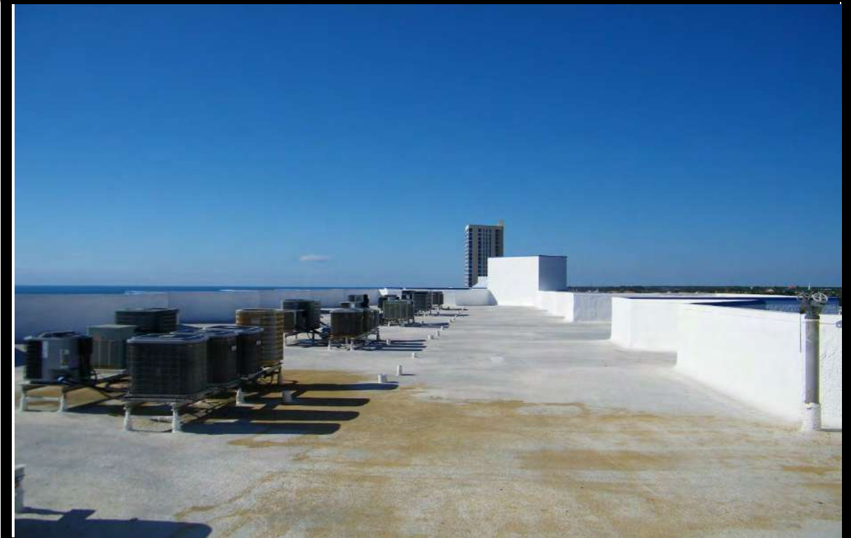
VIEW OF ROOF
