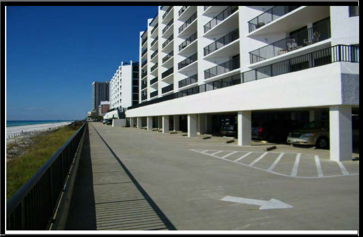
VIEW OF TYPICAL BUILDING COMMON AREAS
