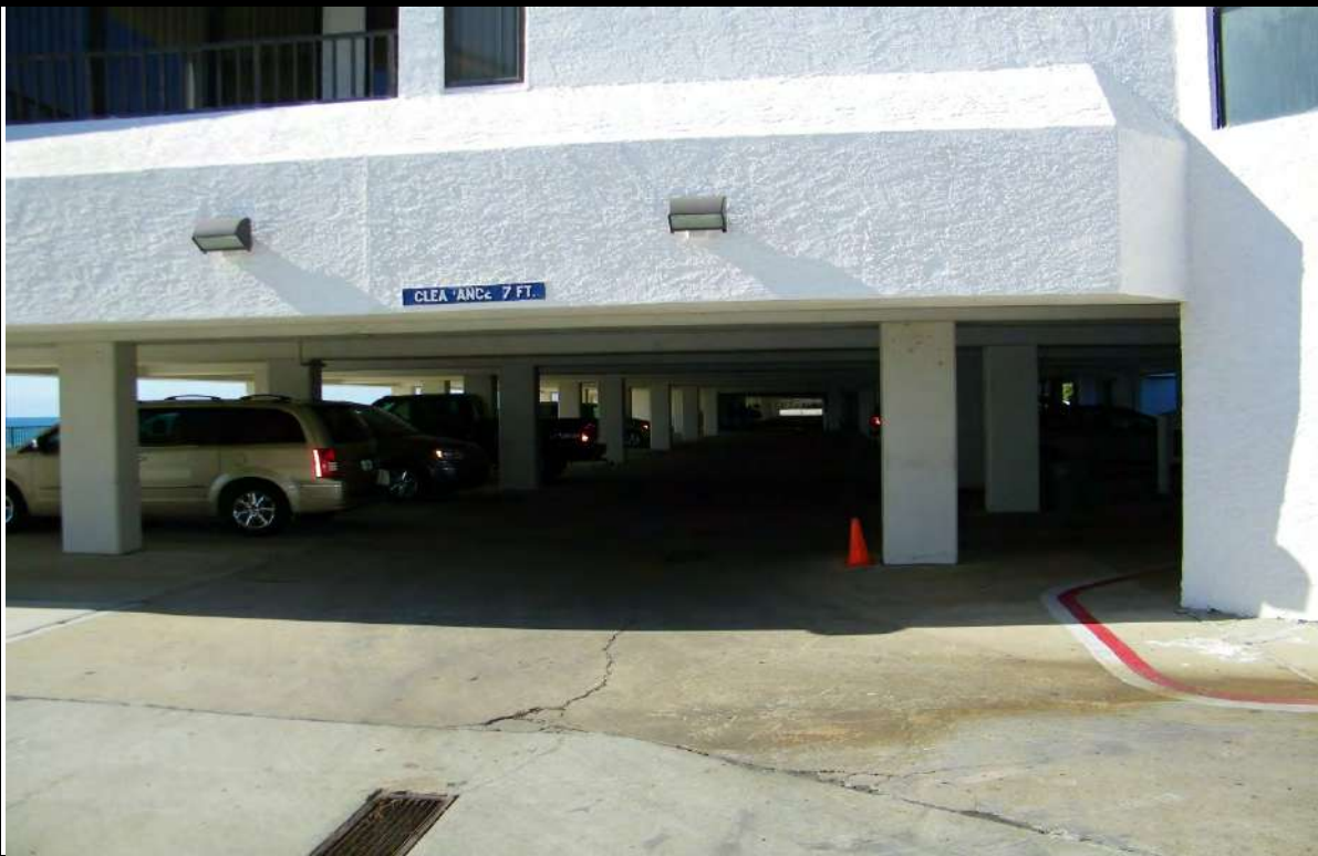
VIEW OF TYPICAL BUILDING COMMON AREAS
