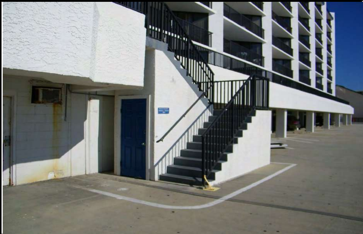
VIEW OF TYPICAL BUILDING COMMON AREAS
