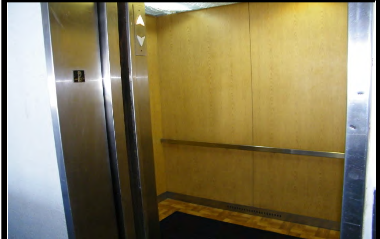
VIEW OF TYPICAL BUILDING MECHANICAL EQUIPMENT
