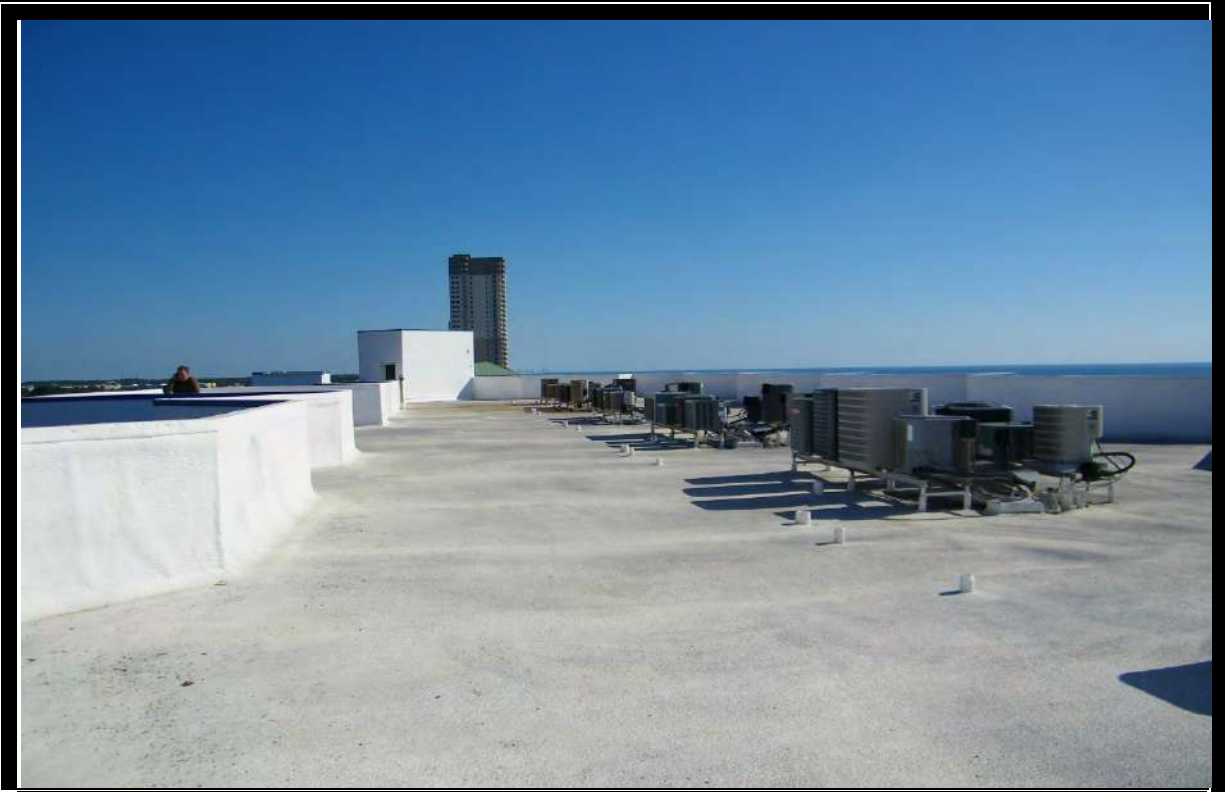
VIEW OF ROOF
