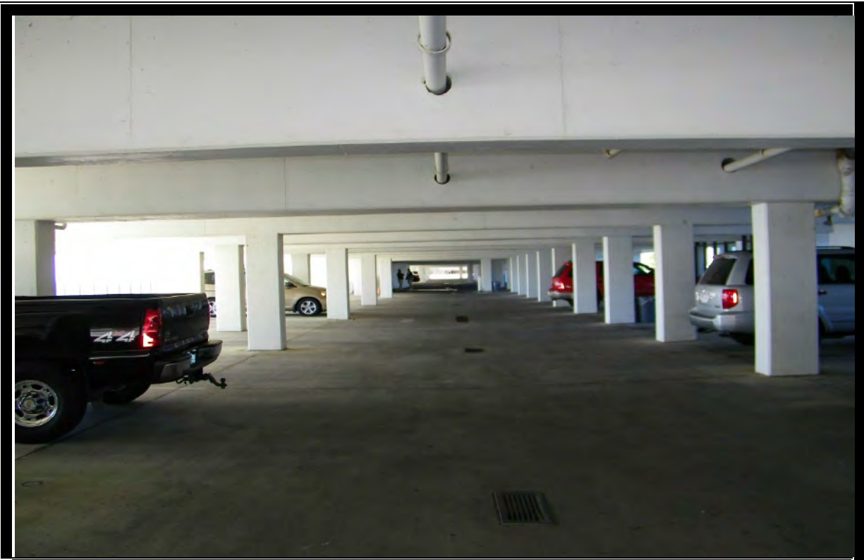
VIEW OF TYPICAL BUILDING COMMON AREAS
