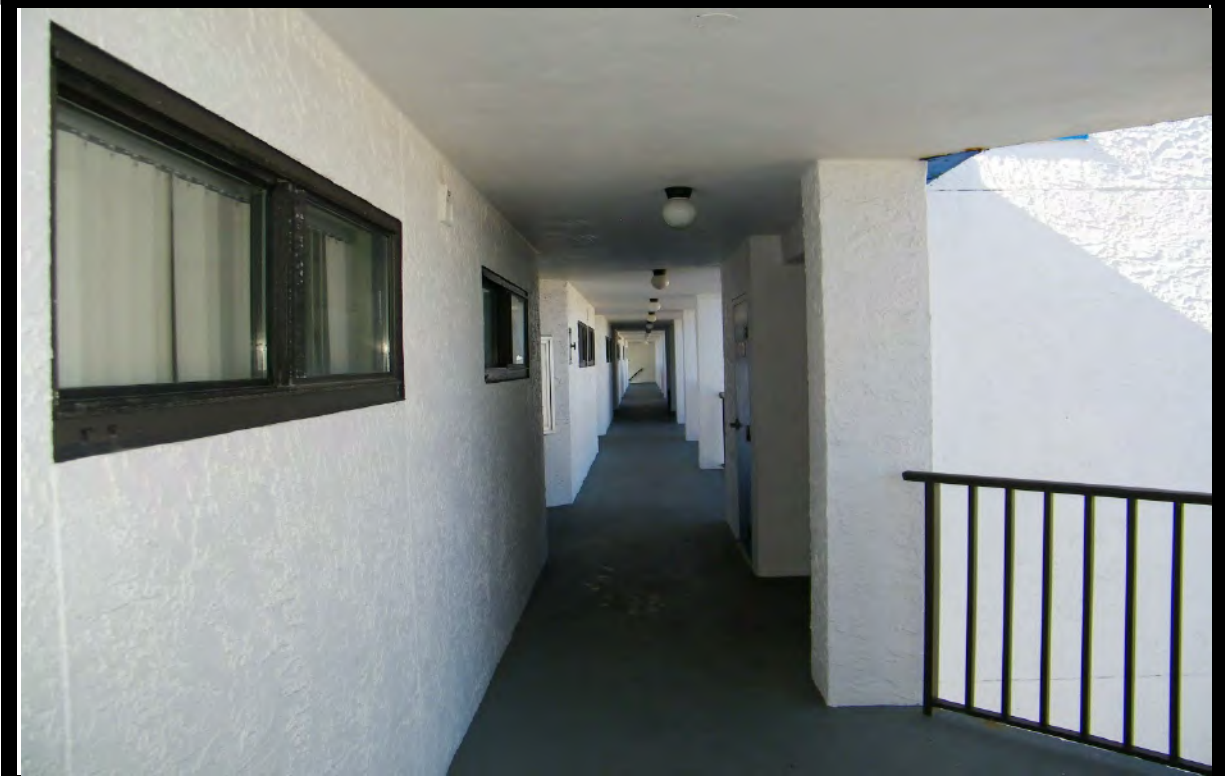
VIEW OF TYPICAL BUILDING COMMON AREAS
