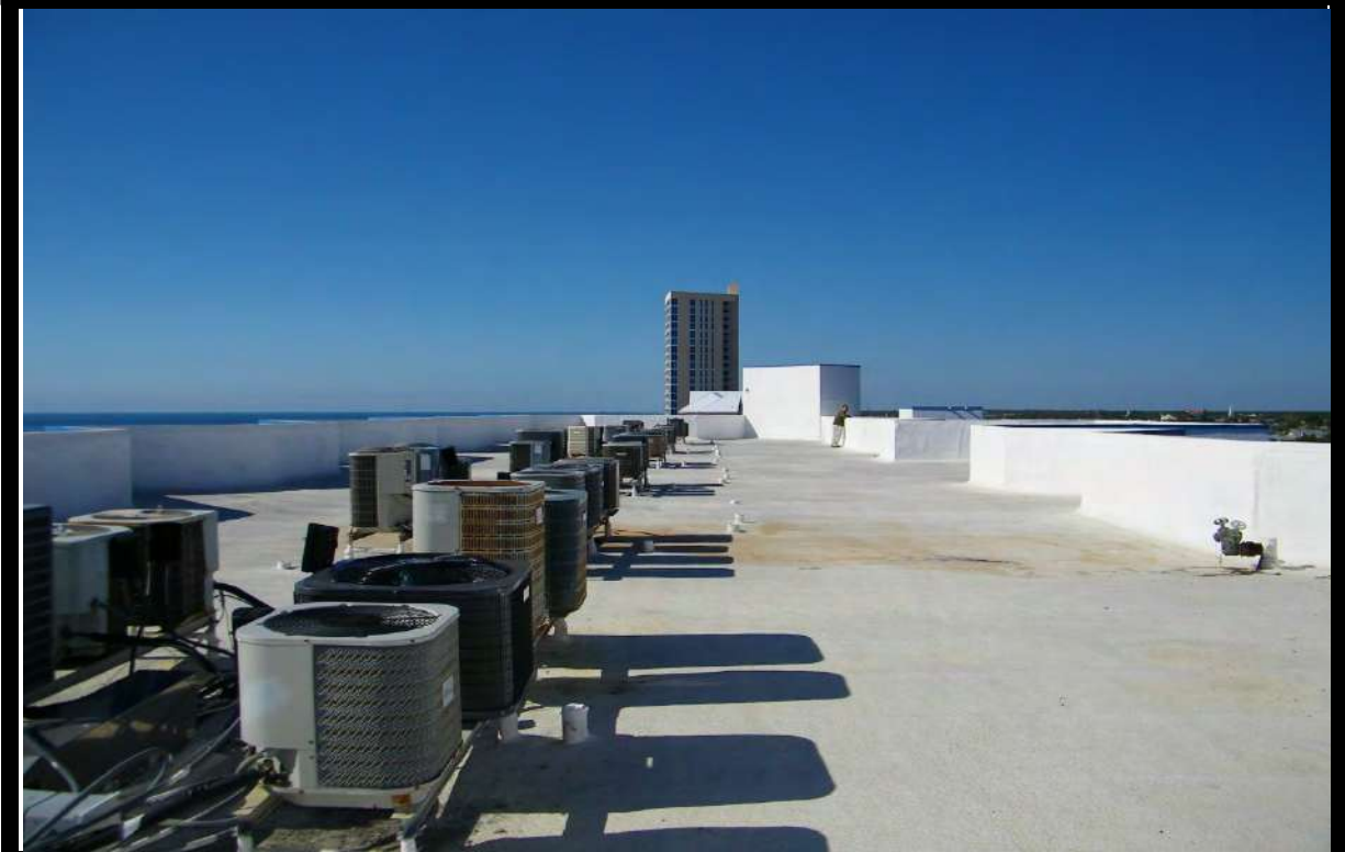
VIEW OF ROOF
