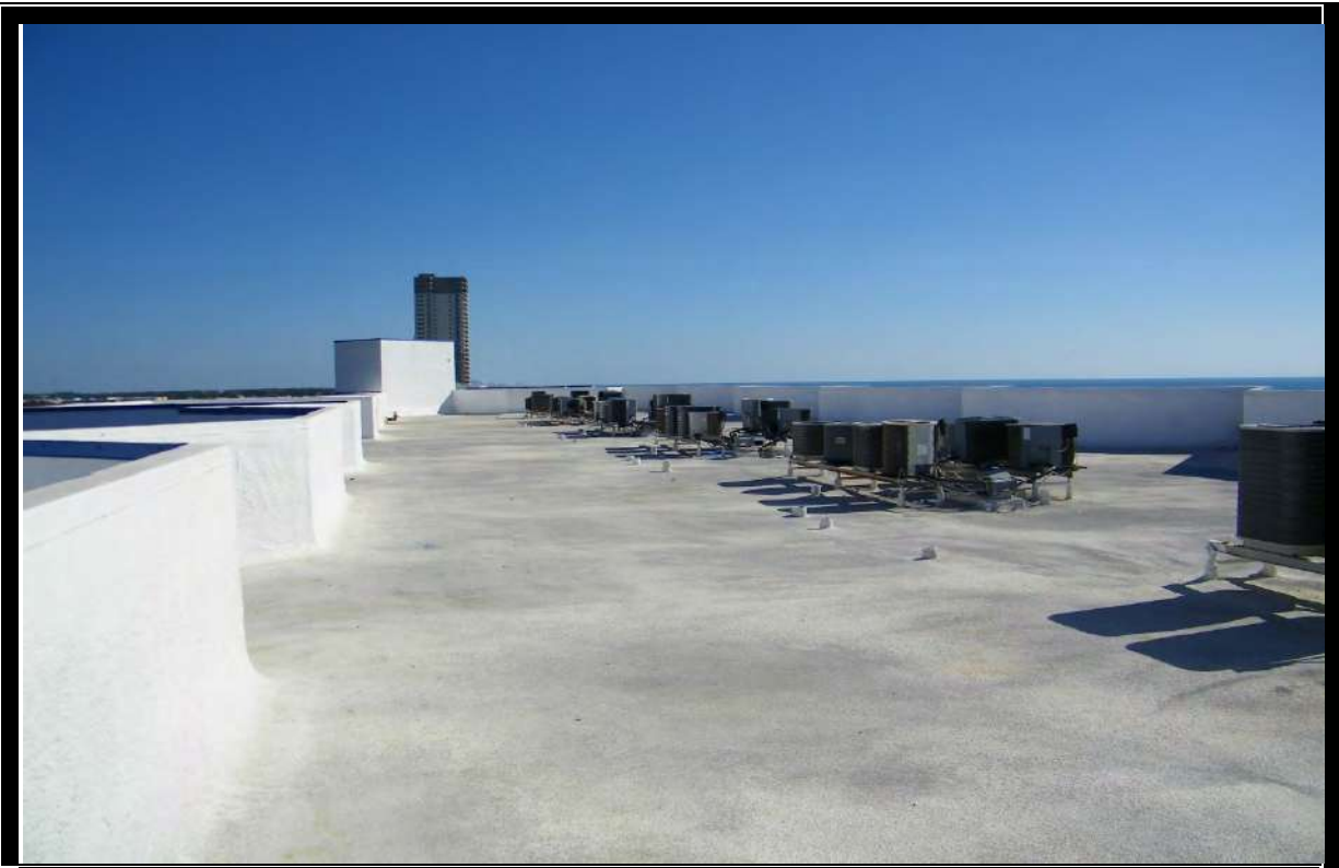
VIEW OF ROOF
