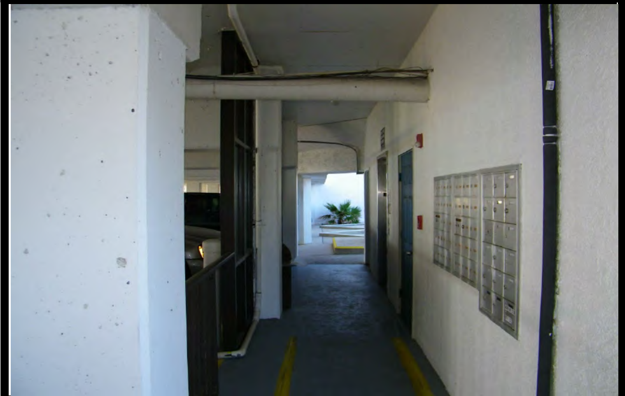
VIEW OF TYPICAL BUILDING COMMON AREAS
